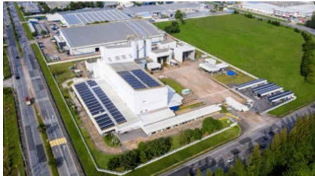
SABIC's sustainability initiatives in Asia also involve reducing the carbon footprint of its operations. At Rayong, Thailand, for example, a 2MW on-site solar farm project generates around a quarter of the plant's energy needs.
