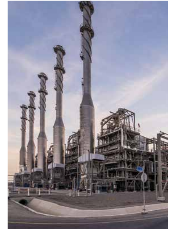
Boilers central to Yansab's Clean Development Mechanism project.
