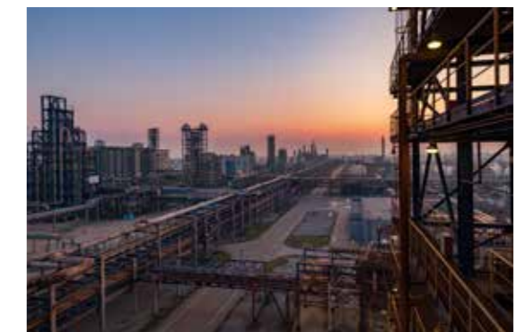
Most of our chemical-production facilities around the world have government-specified limits for air emissions.
