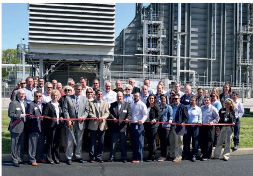
Above: Cogeneration plant at Mt. Vernon, Indiana.
